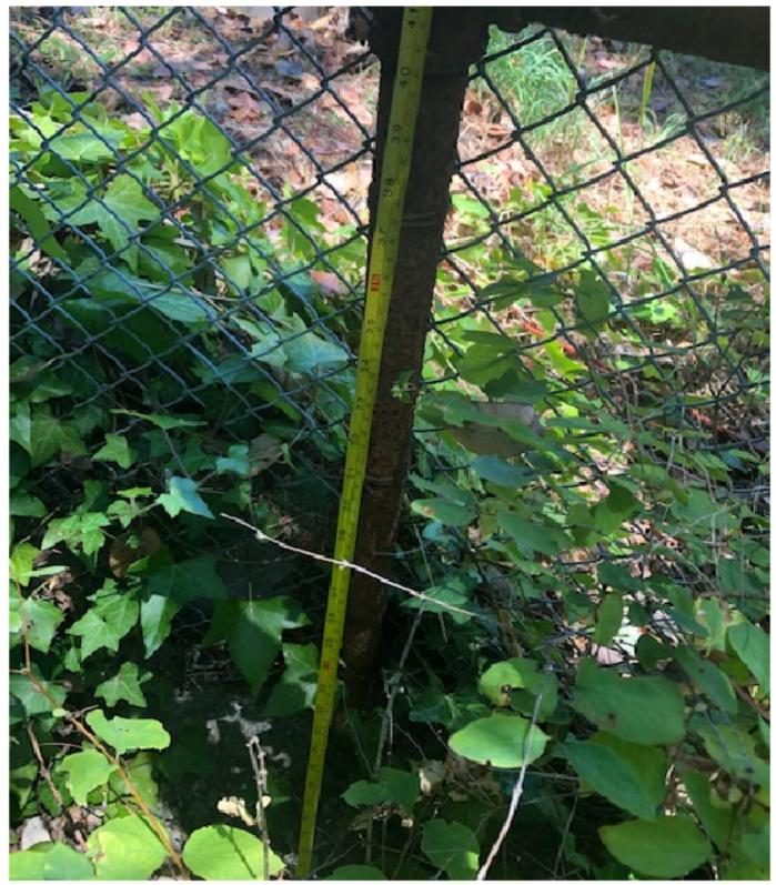
The photograph illustrates that the existing fence is 43 inches high (1.092 meters) from the grade inside the fence and 10 inches high (.0254 meters) from outside grade of fence, the shoulder of the road.
